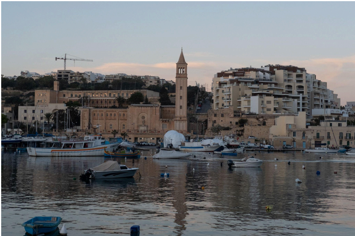
Above: Tower cranes and new “mega projects” show the intensity of development in Marsaskala. Photo: Joanna Demarco.
